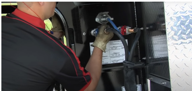
DISCONNECTING AIR/ELEC. LINES
